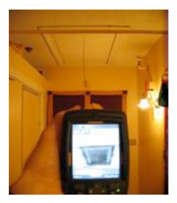
The third floor pull-down stairs demonstrate both air infiltration due to poor air sealing as well as no insulation of the attic stairs. A pliable high quality gasket, and an effective insulating cover are inexpensive and high return on investment improvements in this high stack effect area, if the ceiling of the second floor is to be the uppermost thermal boundary.
