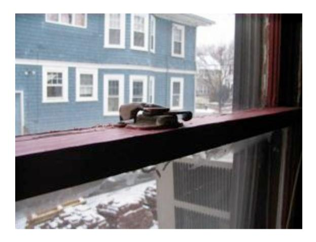
This sash lock was installed backwards, it cannot be used.
