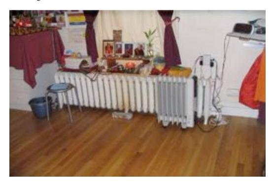
The items on top of the space heating radiator are blocking some of the convection airflow necessary to maximize the heat transfer from the radiator. Removing these items will result in more heat transfer to the room.
