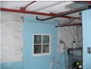
Air leakage around basement door admits a fair amount of cool air into the basement (a high stack pressure area) due to outdoor to indoor temperature driven stack effect.
