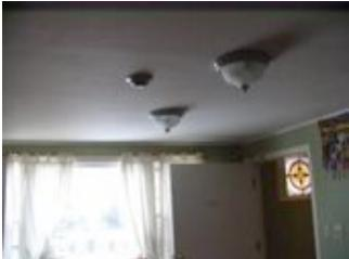
The ceiling lights exhibit the thin, whispy, patterns characteristic of air infiltration.
