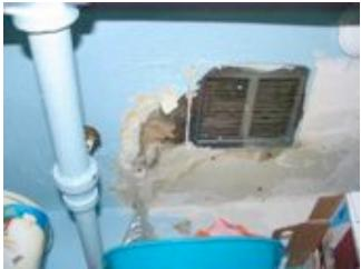
Low temperature air and / or moisture is finding its way into the building, possibly due to the path of the duct connected to this vent. There may also be a correlation to the apparently water induced damage.
