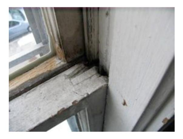
Old wooden windows leak a fair bit of air. This can impact comfort, and does impact energy use, but the energy use significance is frequently exaggerated by window manufacturers.
