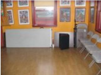
Items blocking baseboards and radiators accelerate heat loss to the outside of the building.
